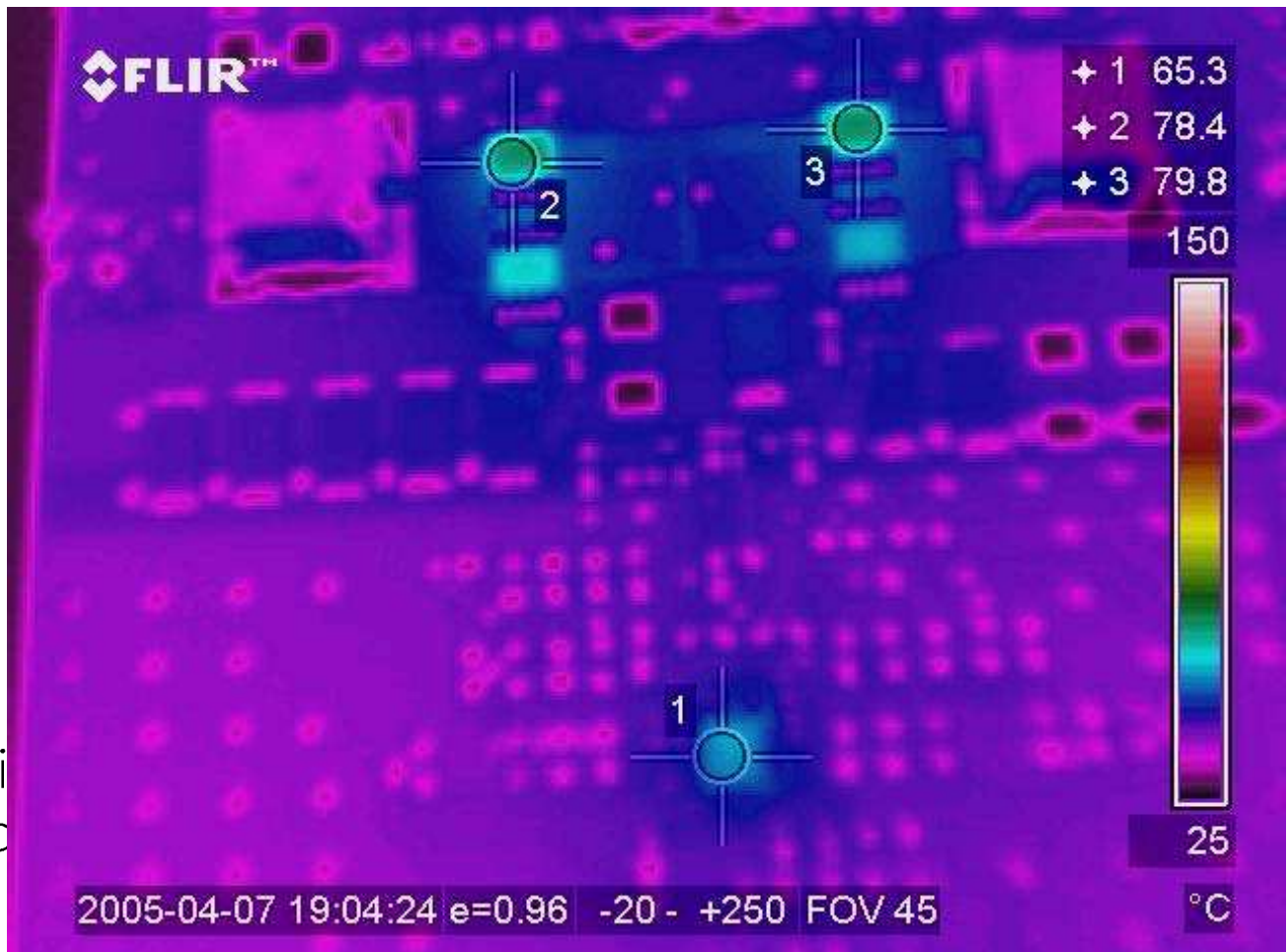
Figure 25- Thermal Images for Both Outputs at Vin:12V, Vout1:2.5V @ 10A, Vout2:1.8V @ 10A. Room Temperature, No Air Flow
